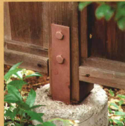
Heavy-duty post bases are excellent foundations for fences. The steel pad under the post is raised slightly above the concrete to keep the post dry. Grout between the steel pad and the concrete ensures good bearing.
